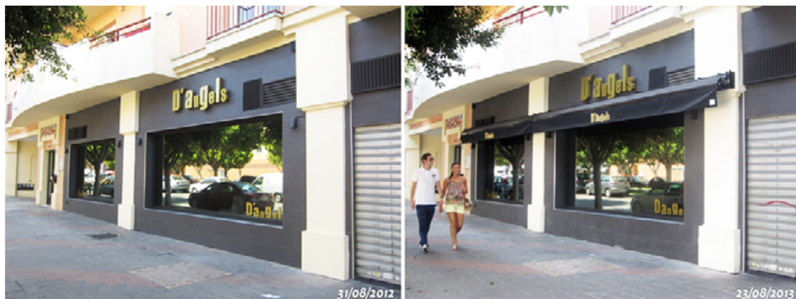
Figure 9. Installation of new awnings at entertainment venues.
